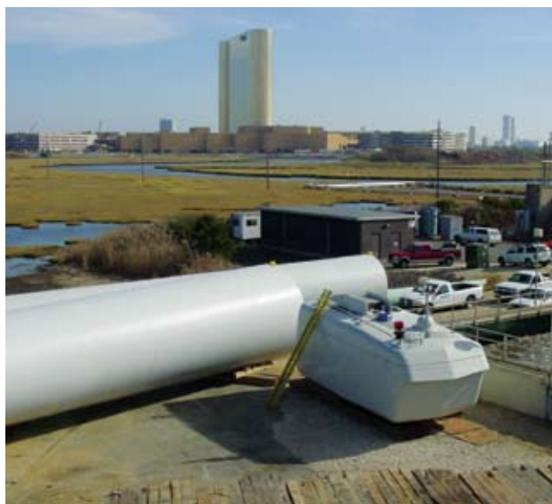
A work in progress. The Jersey-Atlantic Wind Farm was fully operational January 1, 2006. Each 1.5 megawatt turbine is 262 feet high and the blades are 120 feet long. The total height from the bottom of the tower to the tip of the blade is more than 380 feet, about the height of a 32-story building.
