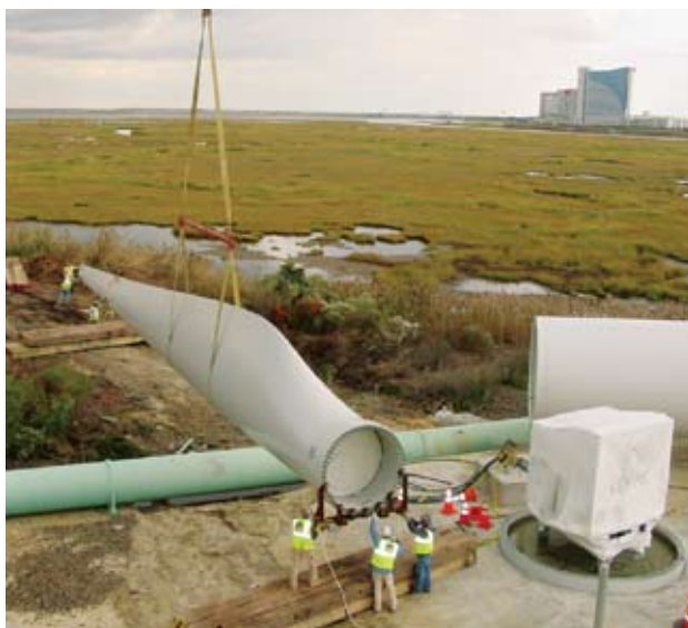
A work in progress. The Jersey-Atlantic Wind Farm was fully operational January 1, 2006. Each 1.5 megawatt turbine is 262 feet high and the blades are 120 feet long. The total height from the bottom of the tower to the tip of the blade is more than 380 feet, about the height of a 32-story building.
